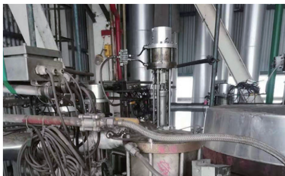
End User: Yunnan Yuntianhua Co., Ltd. Application: SHELL-SCGP Size: NPS 3 Pressure Rating: ANSI Class 900 Inlet Pressure: 7.8MPa Outlet Pressure: 7.8MPa Raw Material: ASTM A182 F316 Fluid: High pressure nitrogen On-line Time: 2012/07/01 Operating Temperature: 250°C Failure Report: None
