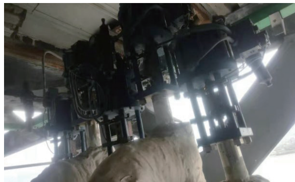
End User: Sichuan Yongxiang Polysilicon Co., Ltd. Application: Polusilicon Filtration Unit Size: NPS 2 Pressure Rating: ANSI Class 600 Inlet Pressure: 9.72MPa Outlet Pressure: 4.2MPa Raw Material: ASTM A182 F316L Fluid: Hydrogen, HCL, chlorosilane On-line Time: 2018/06/01 Operating Temperature: 250°C Failure Report: None
