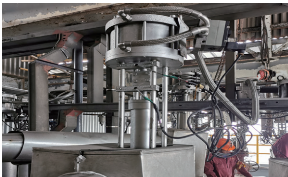
End User: Sinopec Hubei Branch Application: SHELL-SCGP Size: NPS 3 Pressure Rating: ANSI Class 900 Inlet Pressure: 9MPa Outlet Pressure: 3.96MPa Raw Material: ASTM A182 F304SS Fluid: High pressure nitrogen On-line Time: 2015/05/01 Operating Temperature: 250°C Failure Report: None
