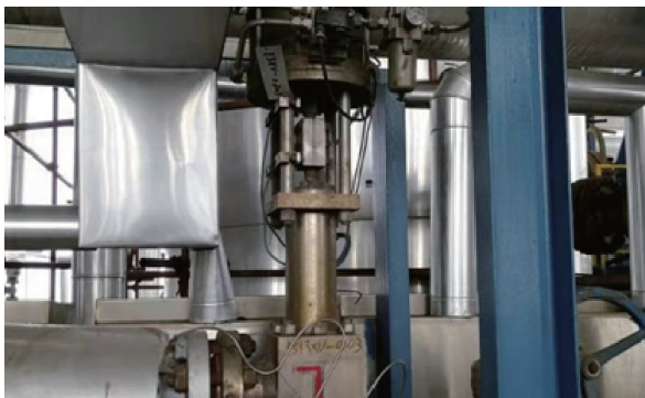
End User: CNOOC Huizhou Petrochemical Co., Ltd. Application: EGAS Filtration Unit Size: NPS 3 Pressure Rating: ANSI Class 1500 Inlet Pressure: 9.72MPa Outlet Pressure: 4.2MPa Raw Material: ASTM A182 F316L Fluid: Syngas On-line Time: 2018/06/15 Operating Temperature: 275°C Failure Report: None
