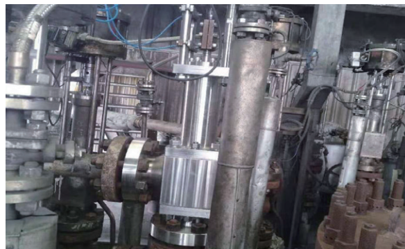
End User: Yunnan Dawei Ammonia Co., Ltd. Application: SHELL-SCGP Size: NPS 3 Pressure Rating: ANSI Class 900 Raw Material: ASTM A182 F304 Fluid: High pressure nitrogen On-line Time: 2011/03/13 Operating Temperature: 225°C Failure Report: None
