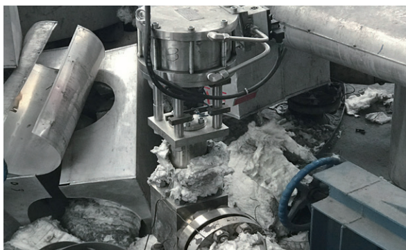
End User: Air Products Lu'an Co., Ltd. Application: SHELL-SCGP Size: NPS 4 Pressure Rating: ANSI Class 900 Inlet Pressure: 9MPa Outlet Pressure: 9MPa Raw Material: ASTM A182 F316 Fluid: Medium syngas On-line Time: 2015/03/10 Operating Temperature: 225°C Failure Report: None
